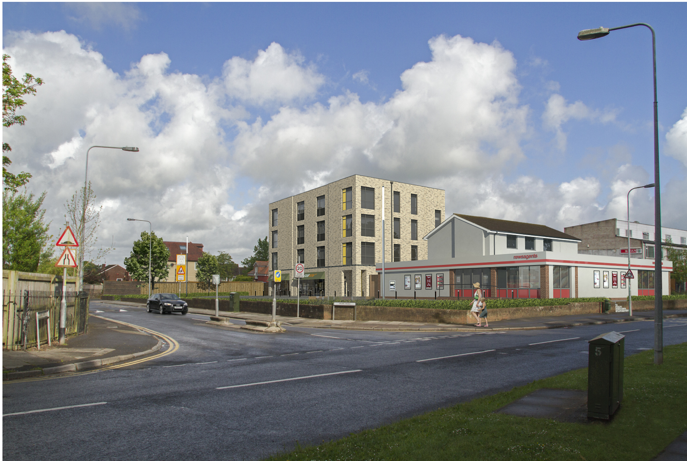
View from South East on Michaelston Road
